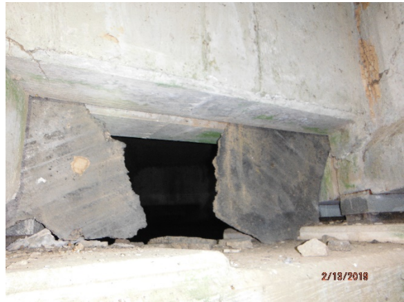
Photo 4. Expansion Joint Board
