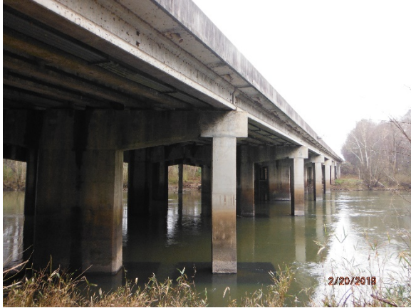
Photo 1. East Side View of Bridge.
