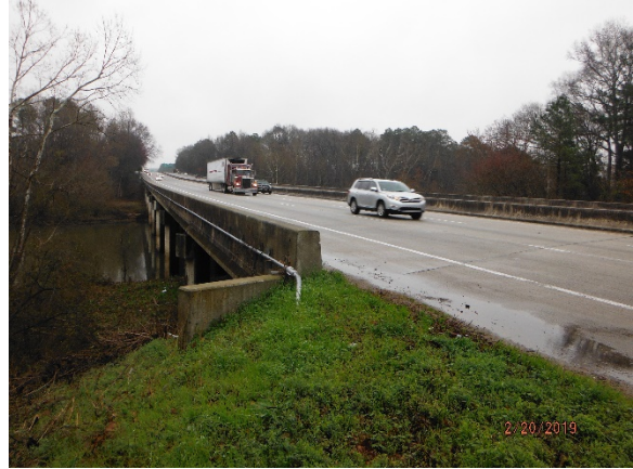
Photo 2. Top of Bridge Deck View.
