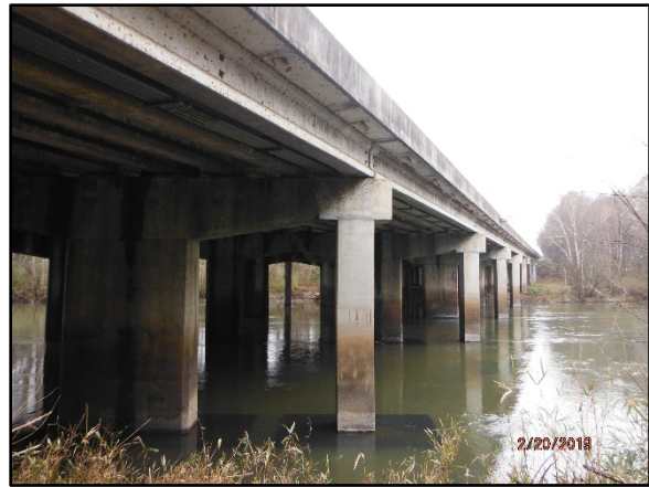
Photo 1 – I-20 Bridge over Saluda River in Lexington, SC.
